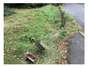
5.4 There are two sets of bollards opposite the cricket pavilion, and the other set further south. Both sets are showing signs of extensive corrosion.
